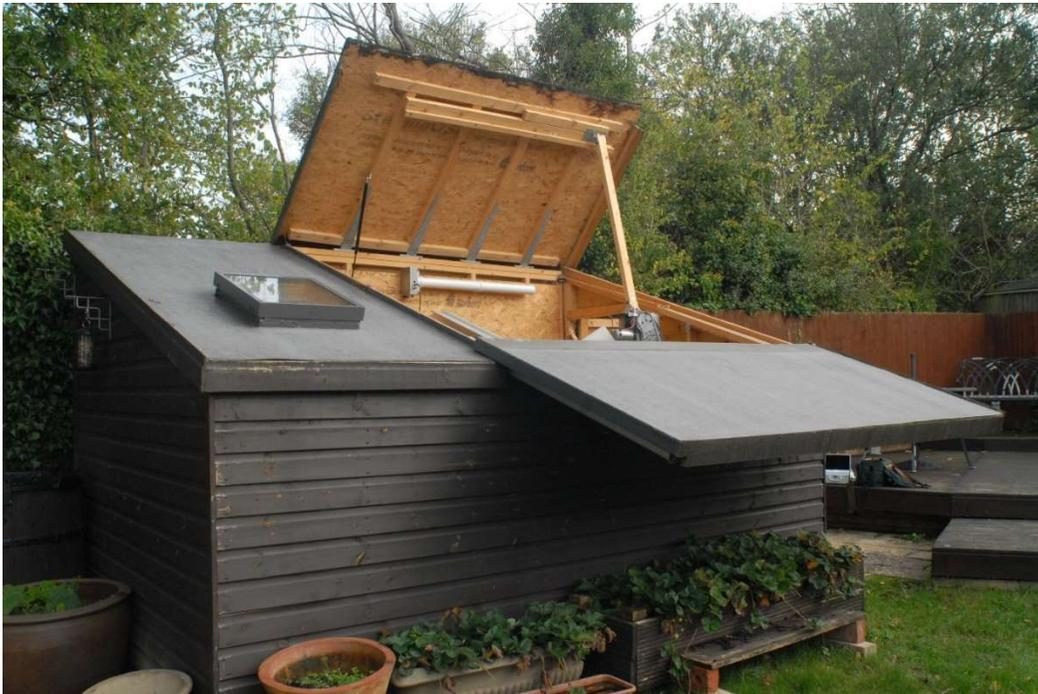
The upper section has proven to be highly effective with there being no visible difference in the light pollution of images taken whilst cars or lorries are passing behind the observatory. The lack of a Northern horizon is a bit of a disadvantage, but the advantages are far outweighed. A roll-off roof design would not have given the protection from the road and would have taken up almost twice the ground area.
