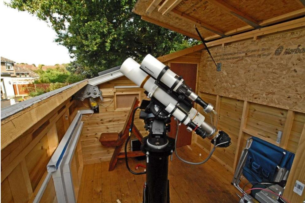
The two cableways are on the left, the upper one carries power circuits and the lower one carries signal cables. (There is a spare piece of trunking lying on the upper trunk way.)
